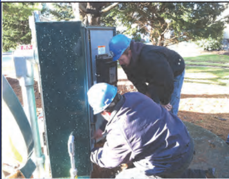
Tom Brosious and Dennis Lloyd work to establish communication from one of South Portland's pump stations.
