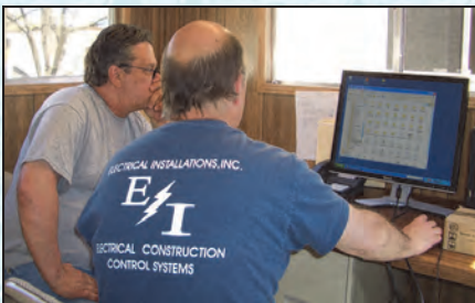
Tom Therrien works with Assistant Superintendent Marty Linstrom as restoration of the plant's control system progresses.
