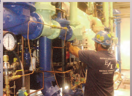
Jake Daku wires valve controls.
